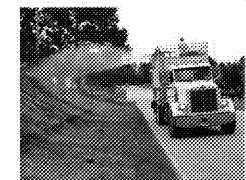
Figure 1. Hydroseeding on disturbed areas
