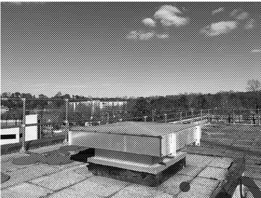
A PICTURE (EXISTING CONDITIONS, FOR REFERENCE ONLY) NTS NOTE: EXISTING HOIST WAY VENT TO BE DEMOLISHED AND REPLACED WITH NEW. REFER TO DETAIL 3/MH601 FOR NEW HOIST WAY VENT AND FLASHING REQUIREMENTS.
